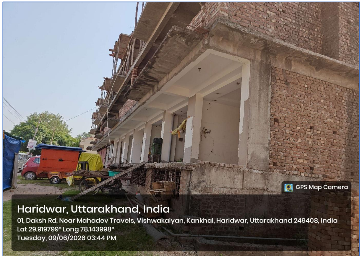
1. Building in question (Basement + 3 Floor).
